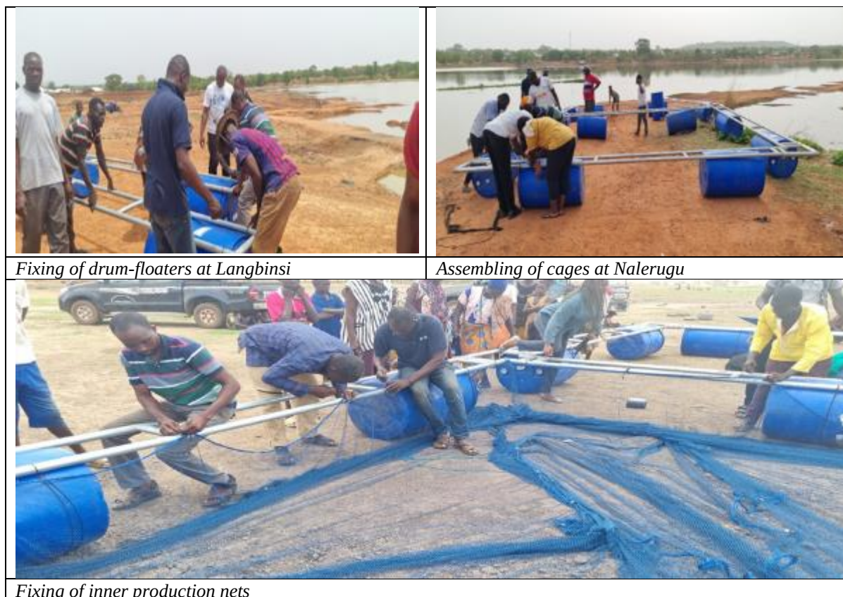
Figure 9. 2: Fixing of Cages in Project Communities
